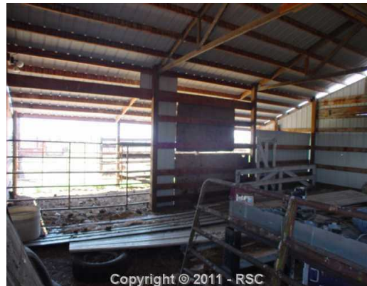
Copyright © 2011 - RSC BARN INTERIOR
